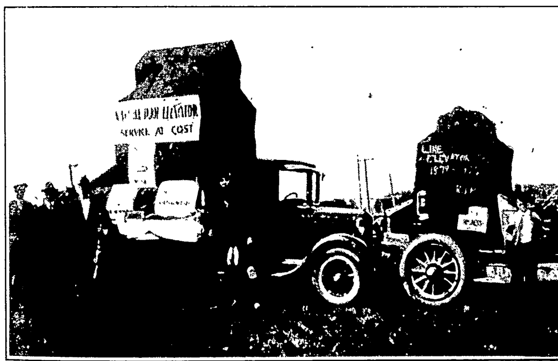
A comparison! New and old elevator systems, as illustrated in floats by the Kaleida Co-operative Elevator Association at Manitou. This display took third prize.
